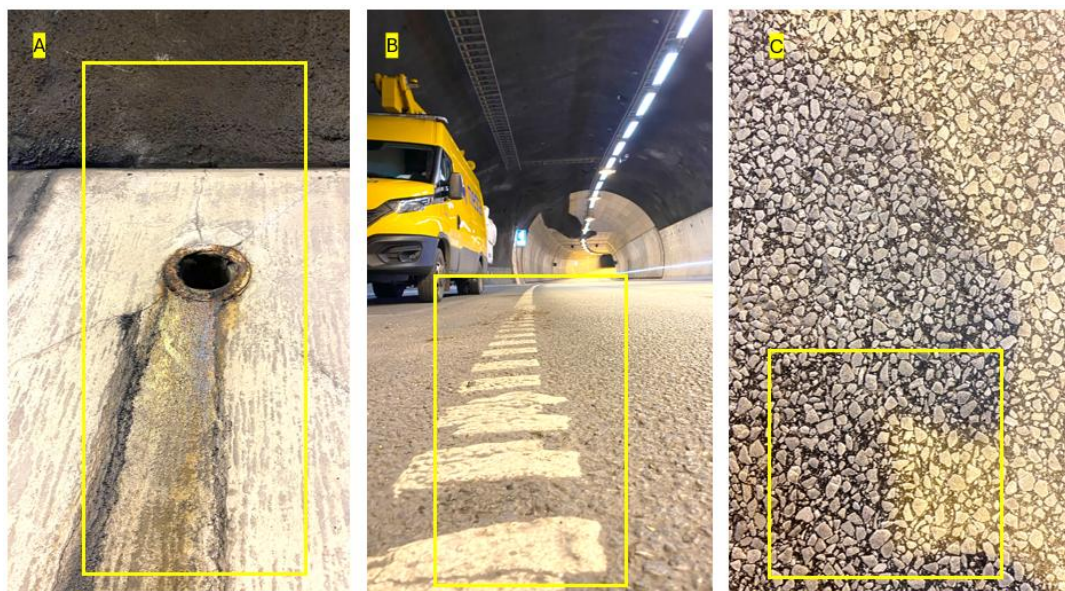
Figure 4: Shows the surface conditions in the Ekeberg Tunnel showing features related to road wear and particle release. A: Corroded steel drainage outlet with dark streaks possibly indicating runoff containing oils or other organic residues. B: Worn thermoplastic road markings showing abrasion, a potential source of road associated microplastic particles. C: Exposed road aggregate (road skeleton) where the bitumen binder and finer particles have eroded, illustrating mineral-based road wear particle formation. All images take by Ole Holthusen in the Ekeberg tunnel
