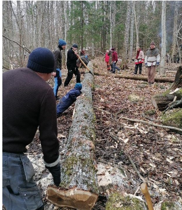
Figure 13, The Meginhufr log is left at 15,5 meters after felling and rotated to be viewed from all angles. Before setting a splitting-line, mumbles and discussion are broken by timely orders to turn every once in a while. Photo by Author.
