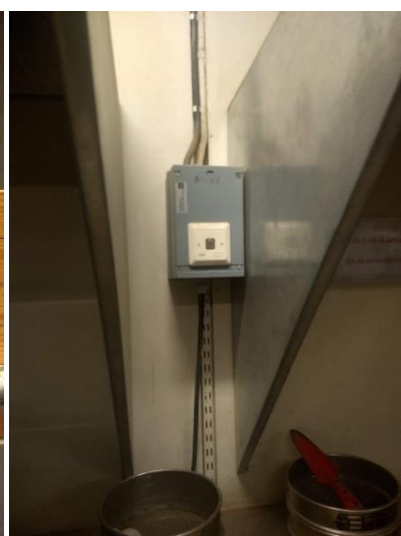
Figure 2.10 – Start button motorized sieve. Photo: Thomas J. Brown (2021).
