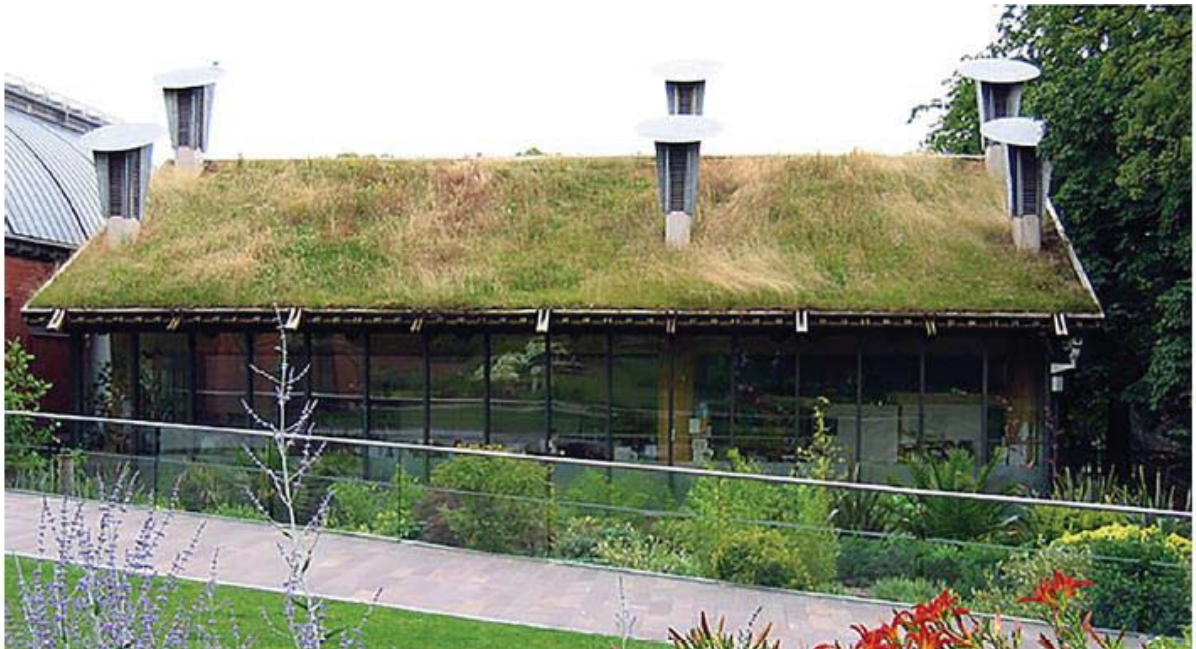
Figure 13. Green roof installed at the Horniman Museum in London (Boano et al., 2019).
