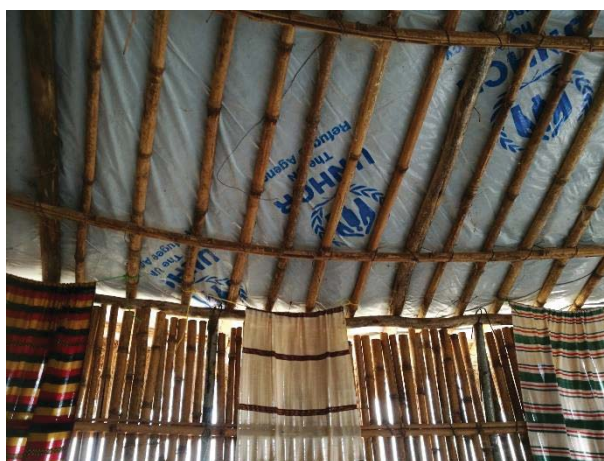
Figure 32: UNHCR sheet used under roof in ARRA office, Photo: Engineers Without Borders
