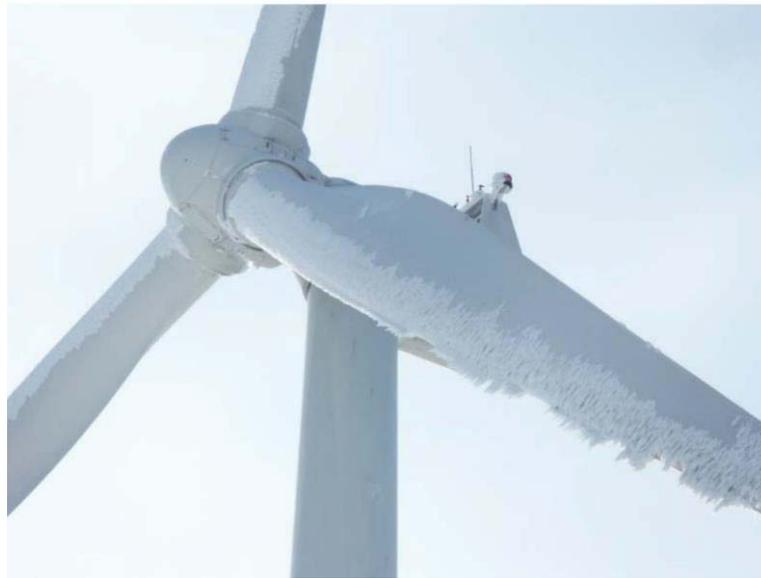
Figure 5: Rime ice on a wind turbine (Ronsten, 2008).
