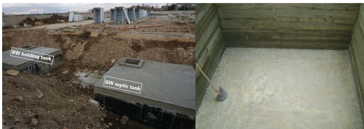
Figure 5.1 (left): The BW holding tank and GW septic tank in Yasmine camp (Photo: NCA, 2016), Figure 5.1 (right): Inside the one-chamber BW holding tank (Photo: IOCC, 2014)
