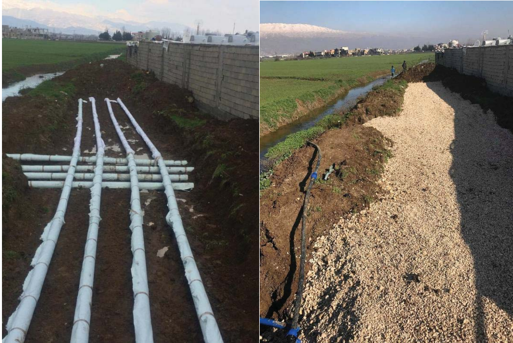
Figure 4.3 (left): The way the pipes cross each other in the soil infiltration trench in Awda camp, Figure 4.3 (right): Backfilling with a layer of gravel over the natural underlying soil and pipes
