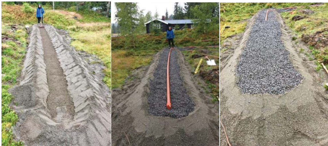
Figure 5.6: Construction of a mound system for a small cabin in Norway (Photos: Petter D. Jenssen)
