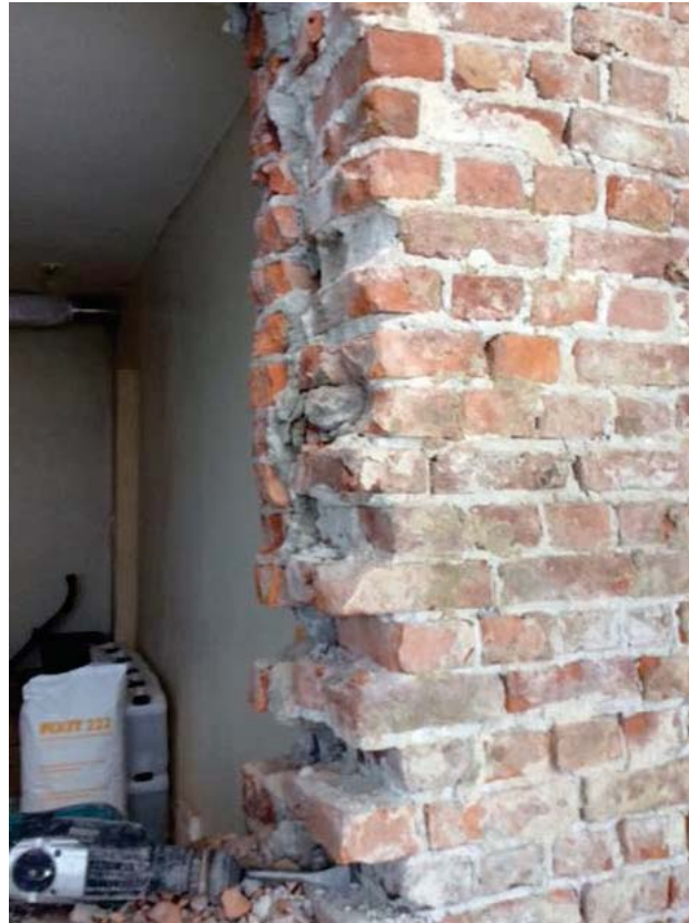
Figure 21 - Picture showing a window cavity after cleaning, before application of FIXIT (source: Boligbygg).
