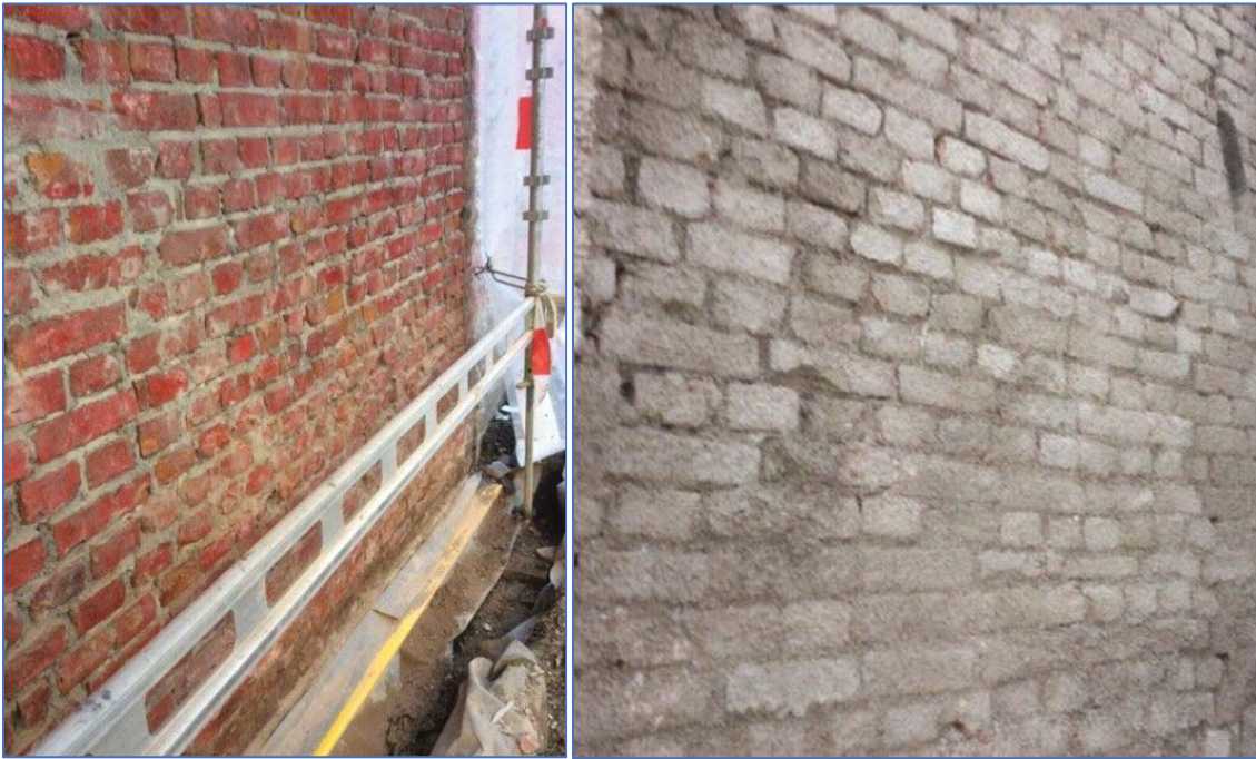
Figure 22- Image one: The clean surface, ready for application of the undercoat layer. Second image: The surface with an undercoat layer. When the undercoat is dry, a layer of Fixit222 can be applied (Source: Boligbygg).
