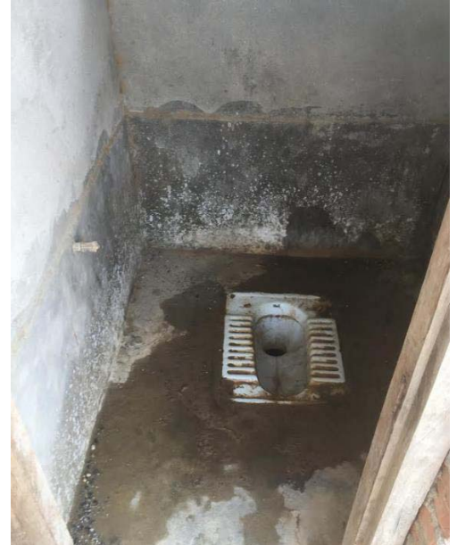
Figure 13. Genderless toilet facility in the middle of the schoolyard on Jana Hit secondary school. Photo Ø.M
