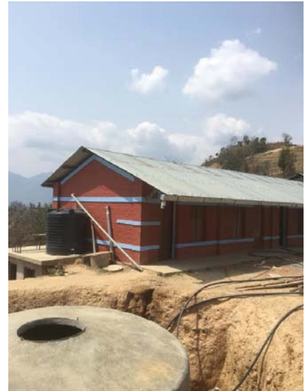
Figure 34. The newly built water storage tank, with a nearby building that easily can exploit the potential for rainwater harvesting. Photo Ø.M.
