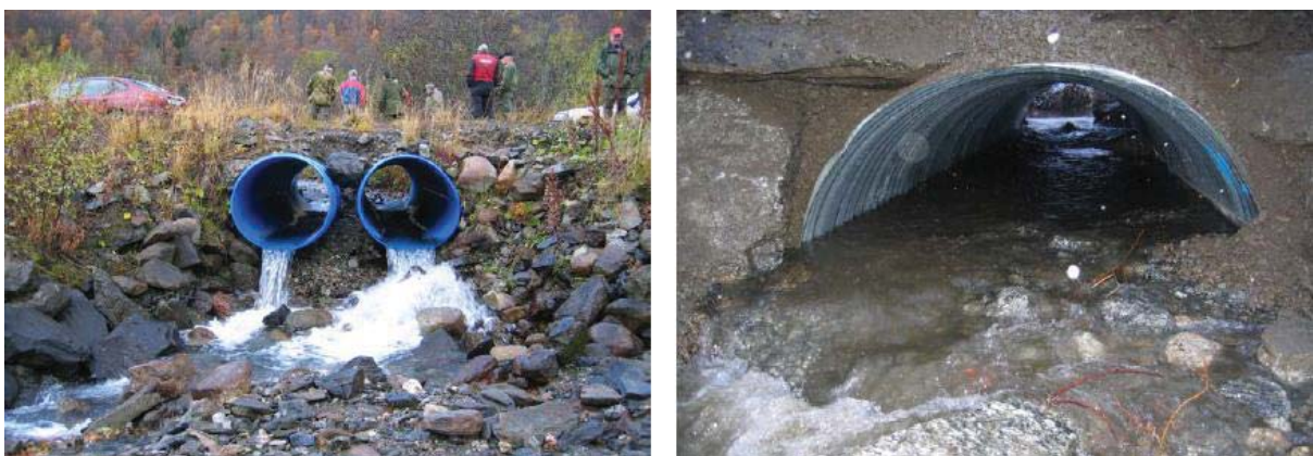
Culvert constructions at Bones; old (left) and new (right). New culvert construction facilitating the movement of organisms between the main river channel and its tributary (Hoseth 2017).
