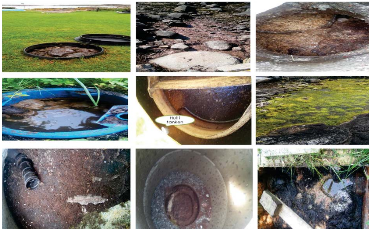
Figure 31: Mosaic picture of some septic tanks and their surroundings in Frøya. Some tanks have holes, the others are filled from sludge due to lack of proper pumping out of sludge and so on. Photo courtesy: Frøya Kommune.
