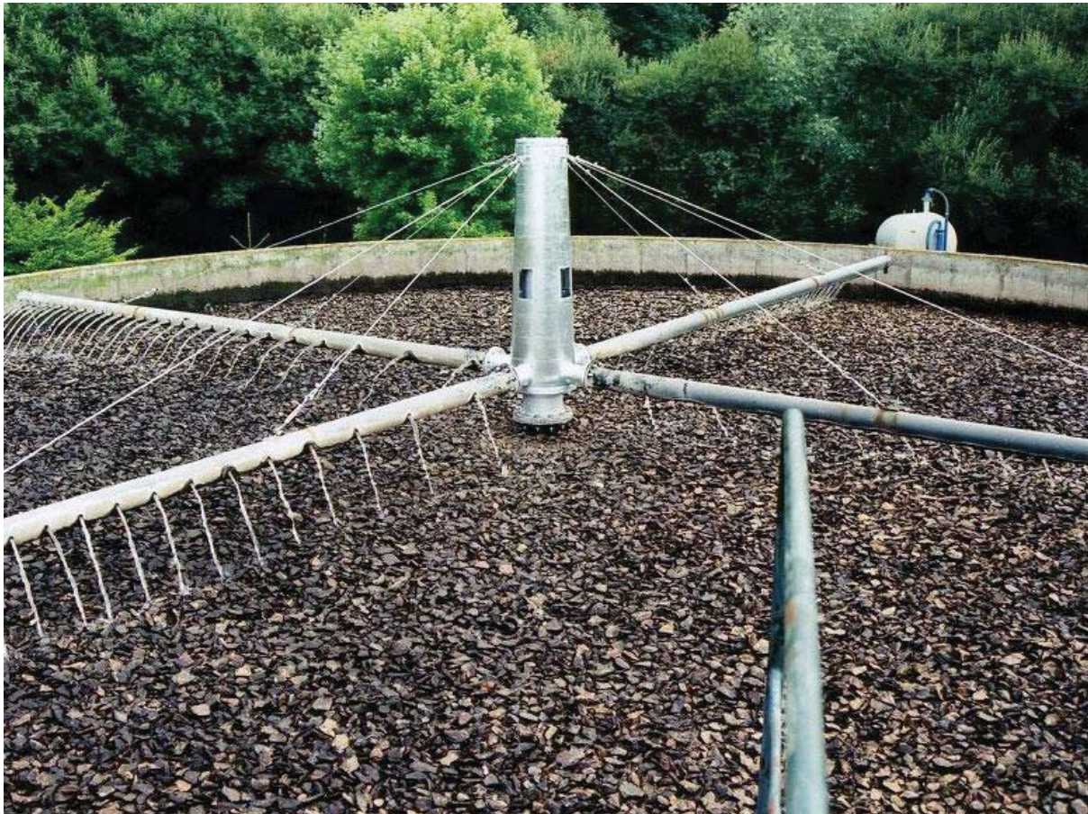
Figure 05: Bio-filter with nozzle for even distribution over the filter material. Picture is taken from (fbprocedes.com).
