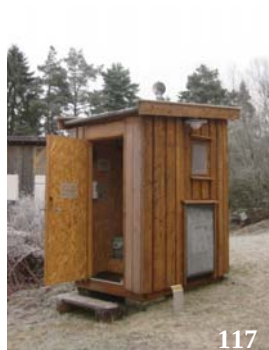
Figure 117: Compost toilet developed in Norway with solar ventilation and dehydration mechanism
