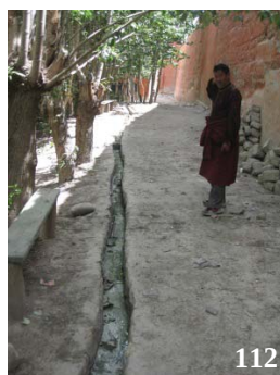
Figure 111: Cemented urinal ditch with clogged drain
