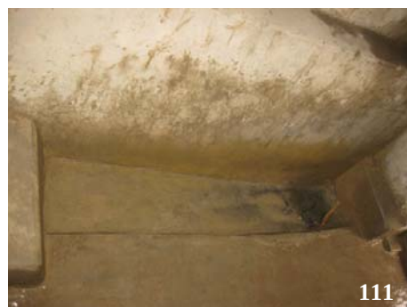
Figure 111: Cemented urinal ditch with clogged drain
