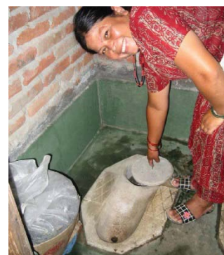
Figure 147: EcoSan toilet with separate collection of urine (front) and feces (back) (WaterAid, 2008a)
