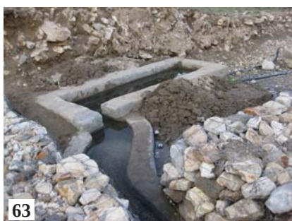
Figure 63: Channel diverting stream water into the intake basin; mound of dug out soil to the right
