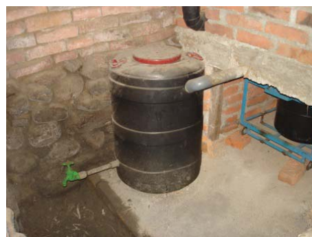
Figure 150: Urine storage barrel with outlet tap (ENPHO, n.d.-e)
