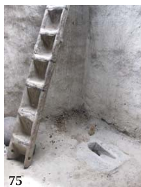
Figure 75: Traditional dry toilet on the second floor, just below the stairway to the roof
