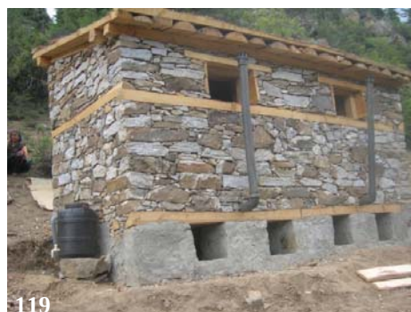
Figure 117: Compost toilet developed in Norway with solar ventilation and dehydration mechanism
