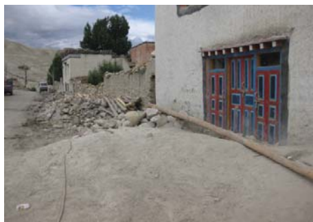
Figure 114: Sand mound covering the Lo Kunphen School's cesspool, just outside the building next to the road
