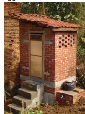
Figure 3: Urine-diverting EcoSan toilet (ENPHO, 2007)
