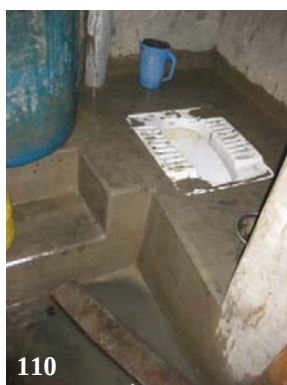
Figure 109: Pour-flush toilet with urinal ditch and toilet chamber behind
