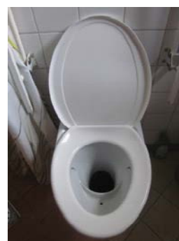
Figure 171: Urine-diverting toilet seat (here in Tingvall, Sweden)
