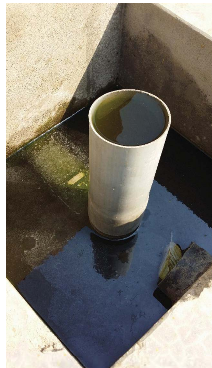
Figure 18: Outlet basin filled with water. The outlet is currently raised to allow the plants to form deeper roots (Photo: Anders Rørå).
