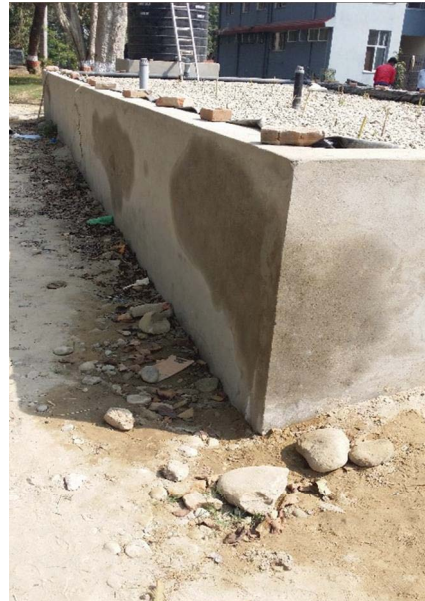
Figure 17: Wet spots on the wall and moist ground indicates leaking from the bed (Photo: Anders Rørå).
