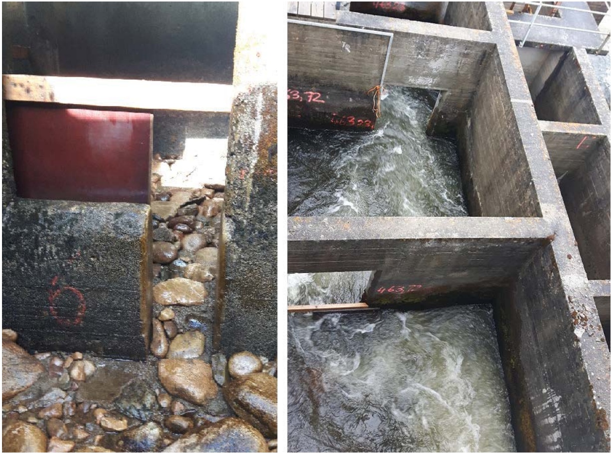
Figure 6 - Left: The new design with 30 cm wide slots and added substrate allow fish to swim along the bottom to ascend the fishway. Right: The picture is showing how it looks in two chambers when the fishway is in operation. Both pictures was taken during the excursion April 10 th , 2017.
