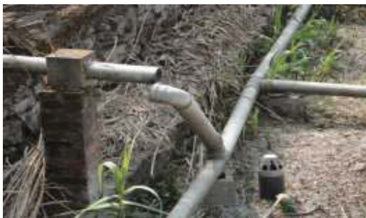
Disconnection of pipe from HFBs
