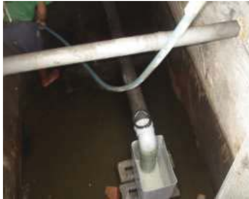
Figure 12: Flushing buckets and intermittent loading system
