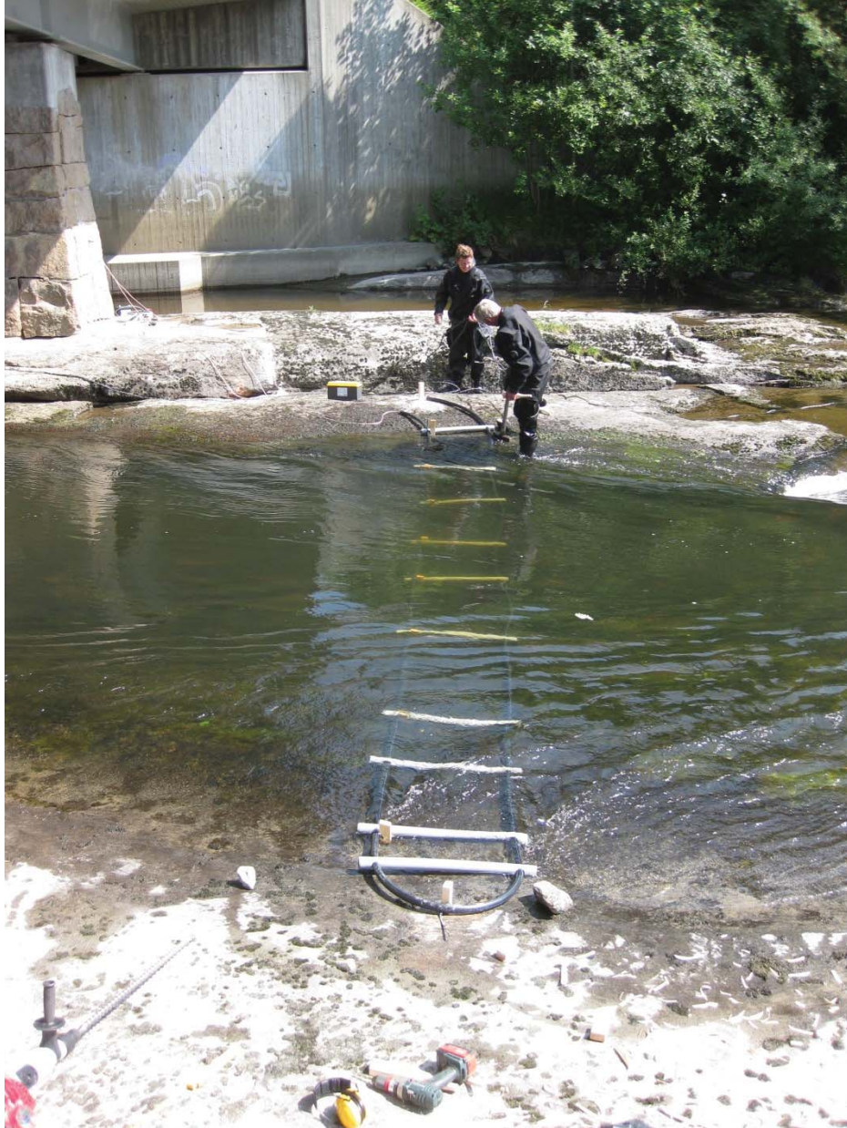
Figure 16. Installation of PIT antenna in Låkedalen.
